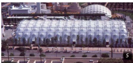
Figure 2: Allianz Arena, Munich: 2.784 pneumatically pre-stressed ETFE cushions.
