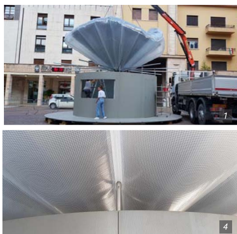
Figure 1. Detail of the installation procedure © Paolo Beccarelli Figure 2a. Plan view and elevation of a single pavilion © Monica Armani Figure 2b. 3D view of a double timber floor slab with two pneumatic roofs © Monica Armani Figure 3. Detail of the FEM structural computer simulations © Maco Technology Figure 4. Detail of the integrated aluminium tubular column © Paolo Beccarelli Figure 5. The Cesare Battisti Square with the pavilions installed © Paolo Beccarelli
